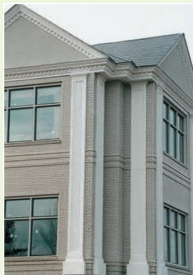
26' Tall Exterior Pilasters
