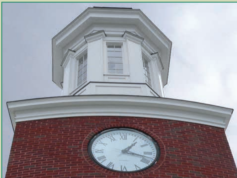
Photo above shows Spectis custom steeple.
